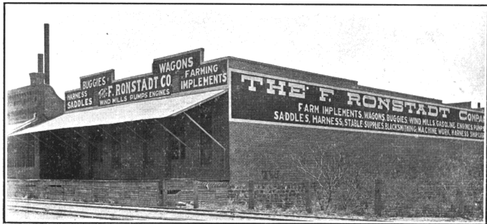
Warehouse on the S. P. R. R. Tracks. Covers area 132 x 148.
